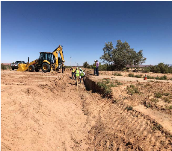
Route N8085 – Many Farms, Arizona; Pipe Installation for Irrigation System
