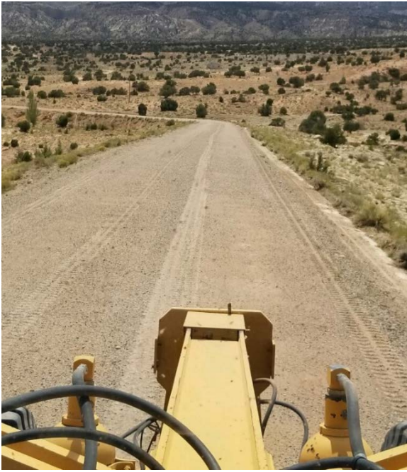
Typical Earth Road Grading in Western Navajo Agency
