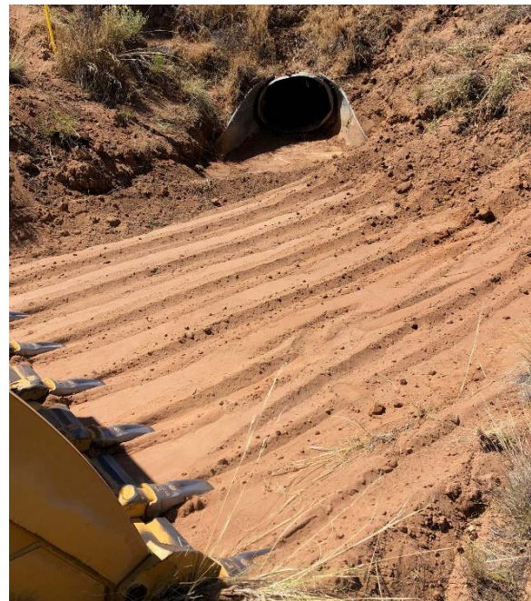
Pipe Cleaned (After)
