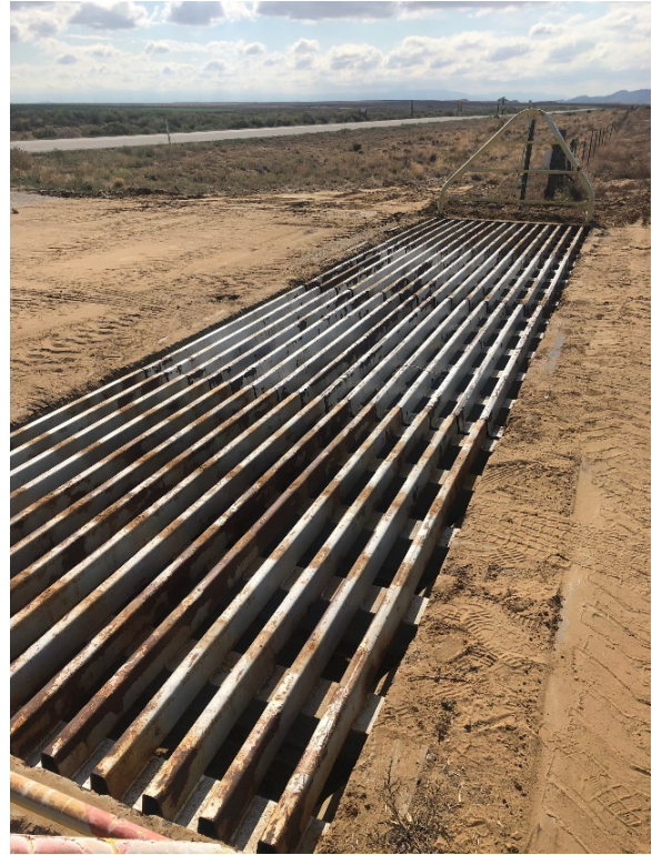
Replaced Cattle Guard Grates & Cleaned
