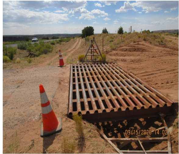
Route N27 – Ganado to Nazlini, Arizona; Fence Repair and Cattle Guard Clean Out
