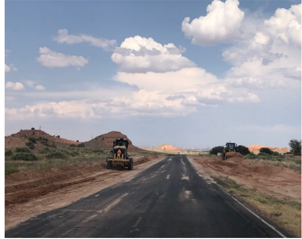
Route N15 – Burnside to Greasewood, Arizona; Silt, Sand, Debris Removal
