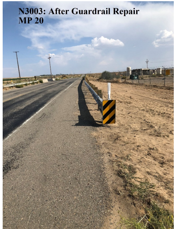
Route N3003 – Guard Rail Repaired (After)
