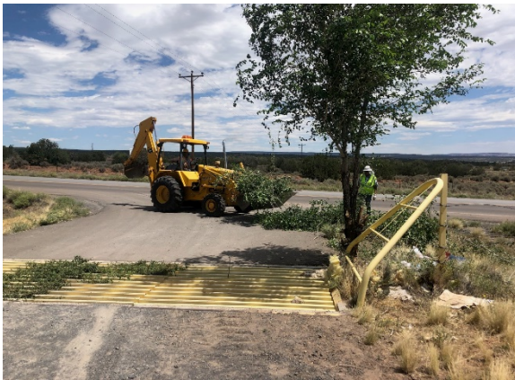
Tree Reducing Sight Distance (Before)
