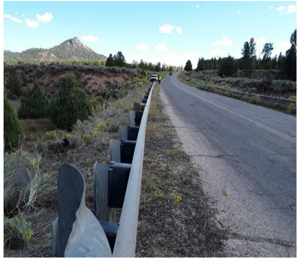
Shrubs/Vegetation Removal on Route N12
