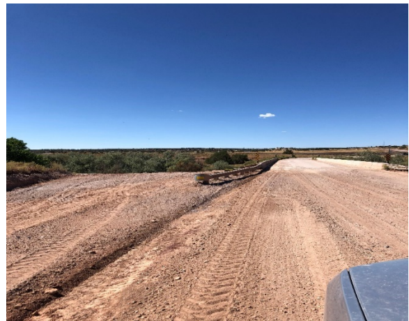
Route N9402 – Allen Town, Arizona; Severe Erosion Gulley and Guardrail Repair
