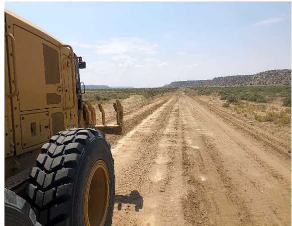
Route N8068 East (Earth Road Grading)
