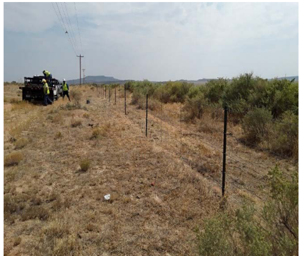
Route N4 – Fence Repair (After)
