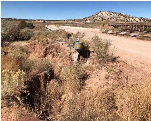
Route N9402 – Allen Town, Arizona; Severe Erosion Gulley and Guardrail Repair
