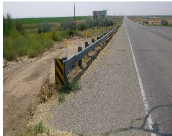
Vegetation Removal along Guard Rail (After)
