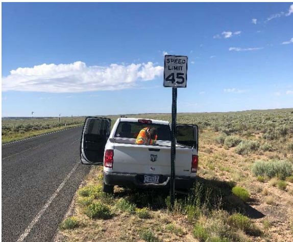
Sign Damage; Bullet Holes (Before)
