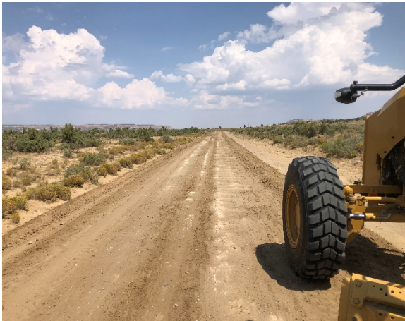
Route N8068 East (Earth Road Grading)
