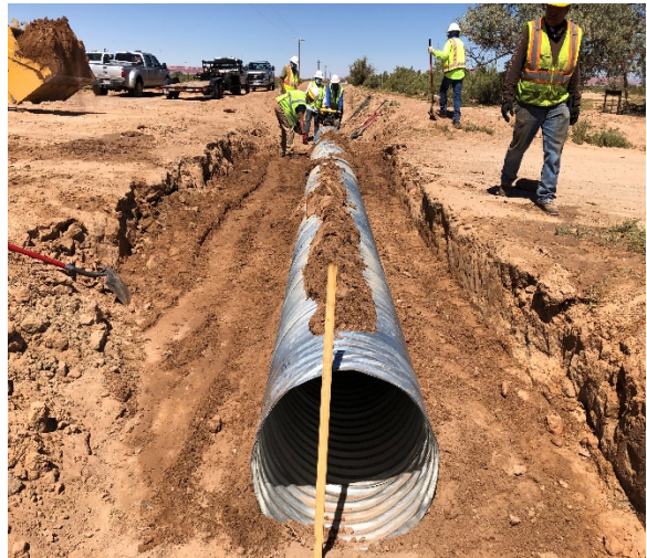
Route N8085 – Many Farms, Arizona; Pipe Installation for Irrigation System
