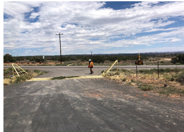
Tree Removed and Guardrail Repair (After)
