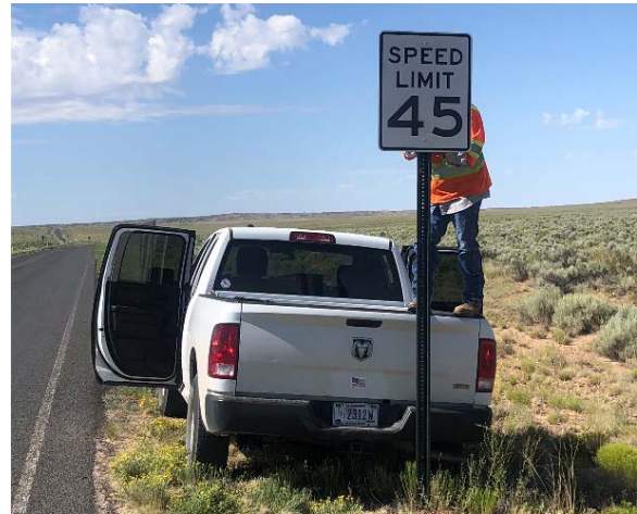
Sign replaced (After)
