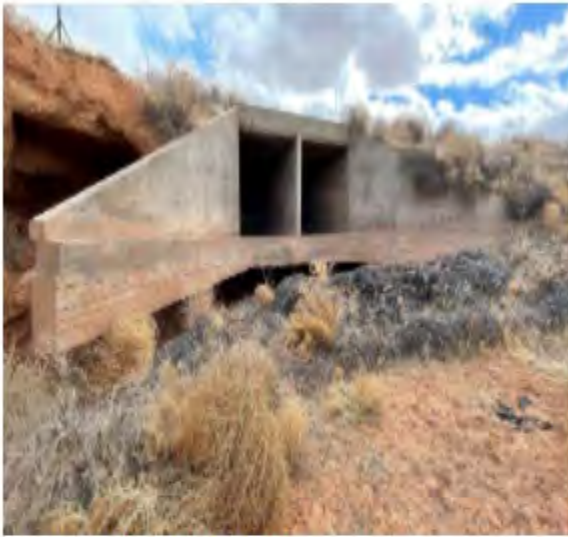
BEFORE: Route N6 CBC: Severe erosion at outlet of CBC.
