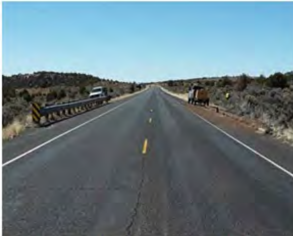
BEFORE: Route N64 - Damaged/Missing Guardrail
