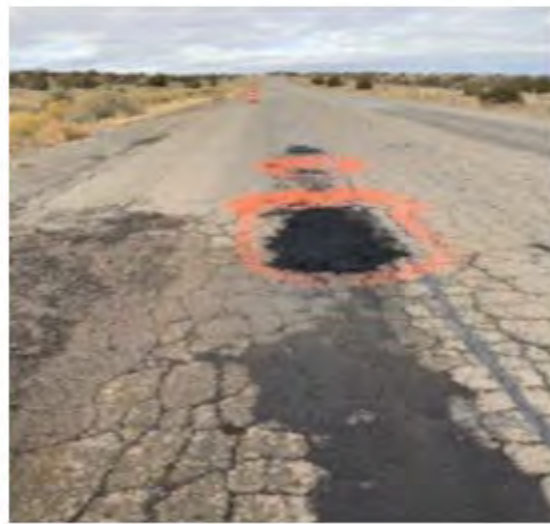
AFTER: Pothole Patching.
