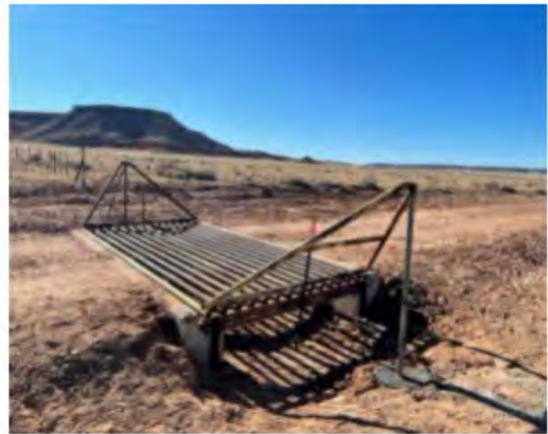
AFTER: Cattleguard installation/repair complete.
