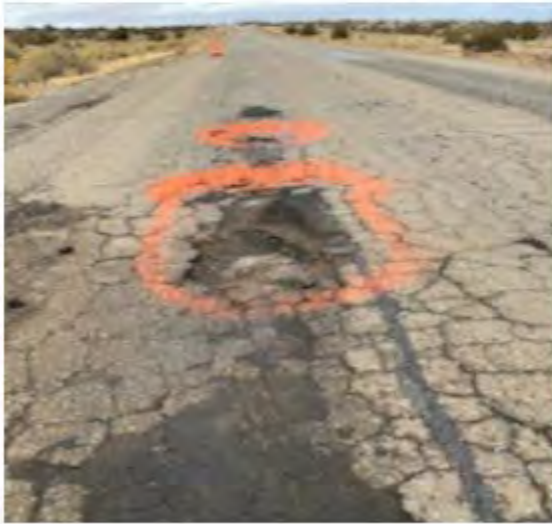
BEFORE: N3003: Damaged Roadway (Potholes).
