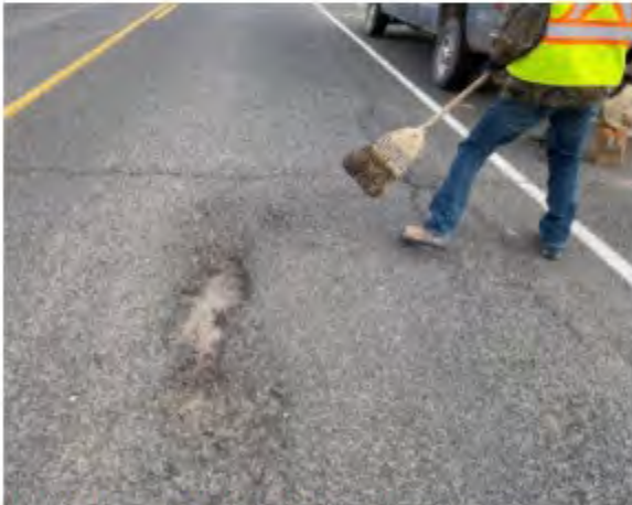
BEFORE: Route N64 - Patching preparation.
