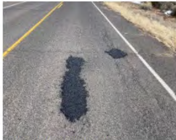
AFTER: Route N64 - Pothole patching
