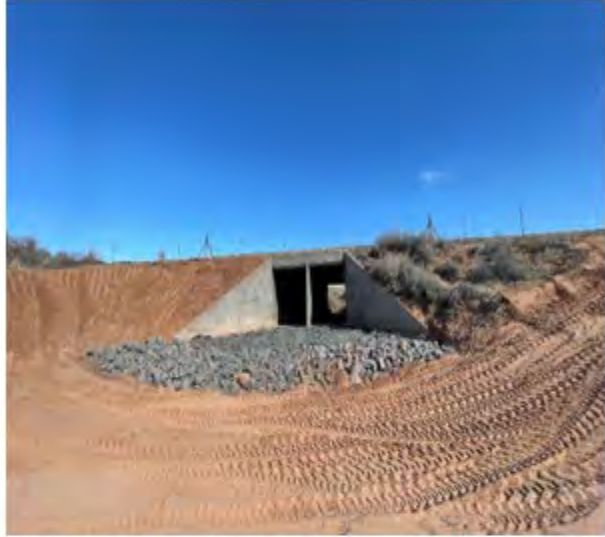
AFTER: Erosion repaired and added more outlet protection
