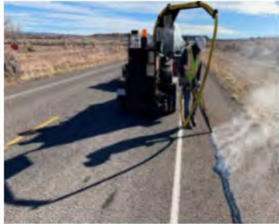
AFTER: Route N27 - Crack Sealing
