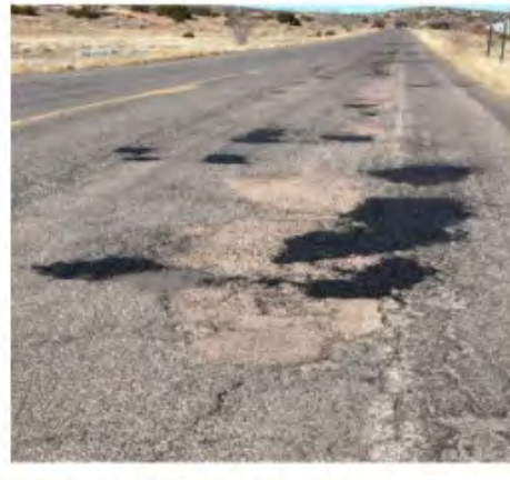
AFTER: Route N112 – Pothole Patching.
