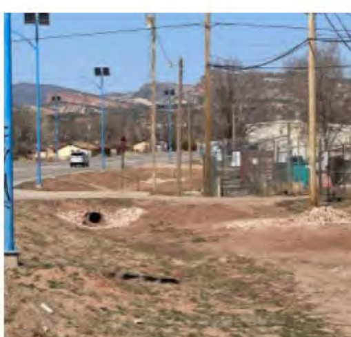
AFTER: Route N12 – Installed riprap at pipe outlet.
