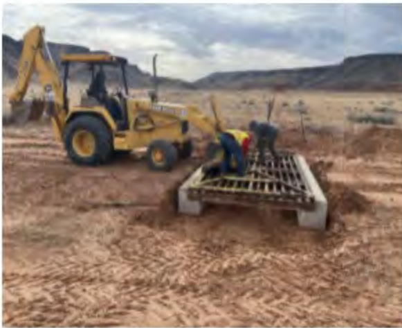
BEFORE: Route N157 – Cattleguard repair in progress.
