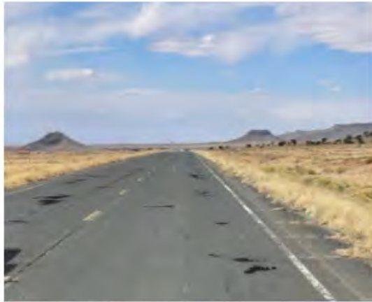
AFTER: Route N15 – Pothole Patching.
