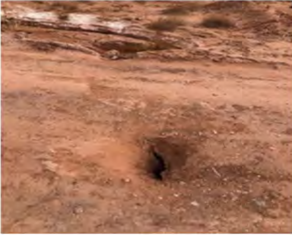
BEFORE: Sign of damaged culvert pipe on WNA road.
