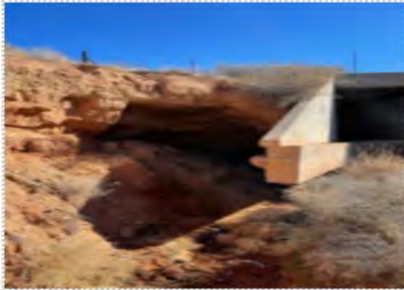
BEFORE: N6 - Erosion Repair under CBC Wingwall
