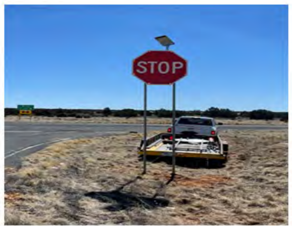
AFTER: NEW LED STOP sign installed.
